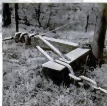
The L-shaped crank at right sends power around a corner
